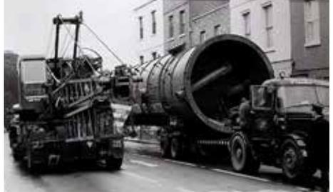
Bear, The Cross and the chicane by the Bell Hotel. Mythe Hill was a real hazard of a runaway hence the two tractors behind to help hold the trailer back.
